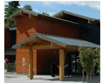
ACRS Office Building
